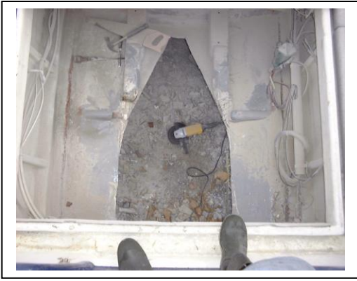
View from inside. Oh my God, there's a big hole in my boat! Next, only a few bits of engine bed to cut out. If only I knew.
