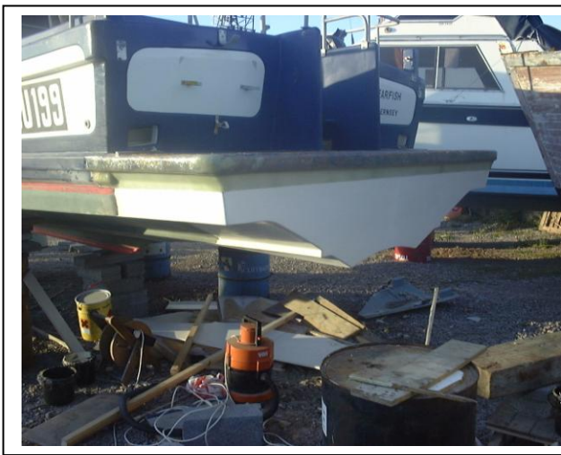
Three coats of 2oz mat overlay the top of the new hull, bonding on to the swim platform and matching the existing structure.
