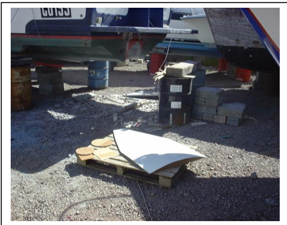
A piece of melamine covered hardboard, cut to shape and waxed, lies near the stern, ready to be fitted as a former (mould).
