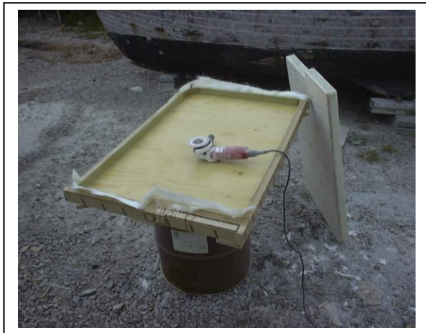
Two of the three new swim platform hatches. Half-inch shuttering ply with a temporary formica/chipboard shutter is glassed 2 x 2oz underneath. After removing the shuttering, 4 x 2oz glass is laid on the top (deck) side.
